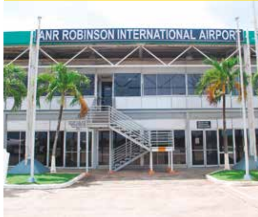
Work on the airport expansion project will commence in 2017
